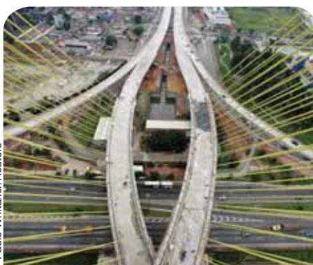
Construction of the Octavio Frias de Oliveira Bridge in São Paulo. Crisis is “stress testing” Latin America.
